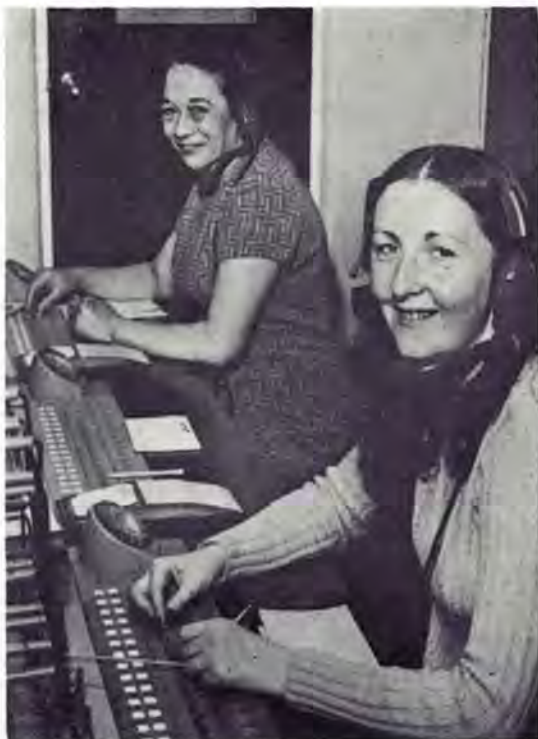
Evelyn and Sue on the North Wirral switchboard.
